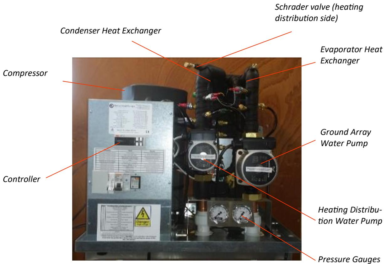
**Fig 3. The internals of a single compressor heat pump**
